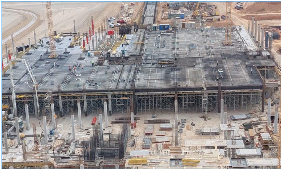
Progress of readiness for departure slab Concreting
