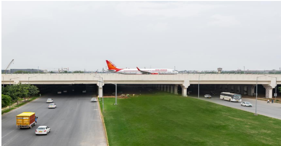
Eastern Cross Taxiway
