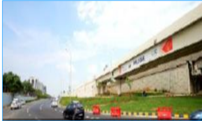
Parallel Access Road Flyover & RE Wall
